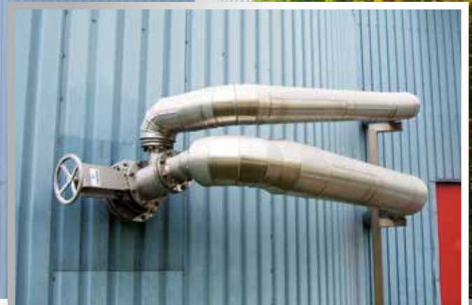
3 water jet air compressors at the 4 000 m 3 clear filtrate storage tank of the paper mill "Blue Paper SAS" in Strasburg. Each water jet air compressor is operated by one circulation pump.
