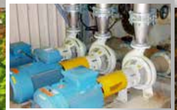
3 water jet air compressors at the 4 000 m 3 clear filtrate storage tank of the paper mill "Blue Paper SAS" in Strasburg. Each water jet air compressor is operated by one circulation pump.
