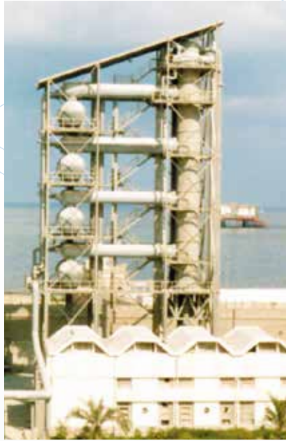
Bridge design with separate steel construction, option of a 2-tower design, 4-stage, cocurrent plant
