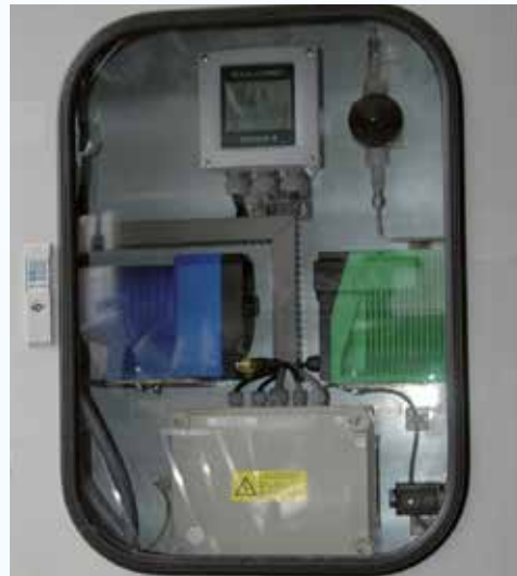
By using a pH-control unit the pH-value of the closed loop water is kept constant.
