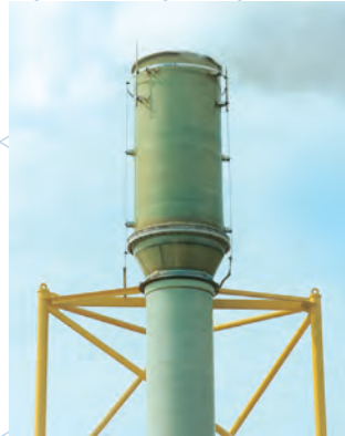
Chimney swirl droplet separator at BASF
