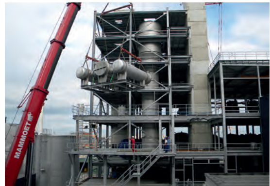
Assembly of an ice condensation block at site
