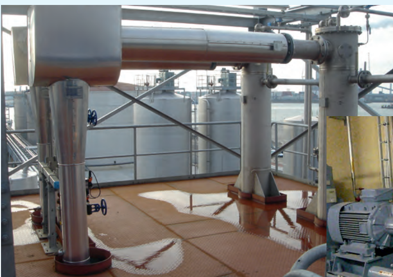
2-stage steam jet vacuum ejectors with shell and tube condenser
