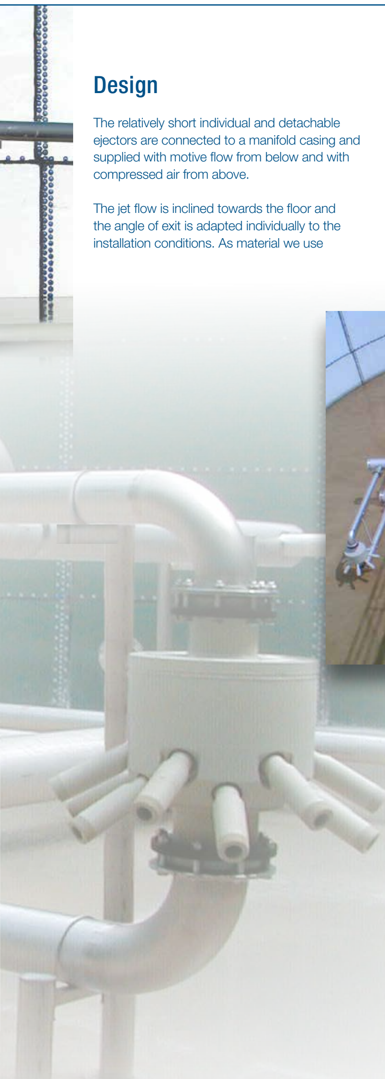
Seven-path ejectors in the 2 000 m 2 aeration tank of a laundry
